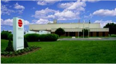
SAN-J Factory in Virginia, USA
