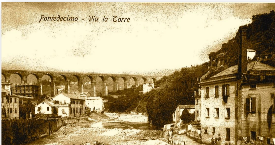
Figure 65. Via La Torre - Pontedecimo
